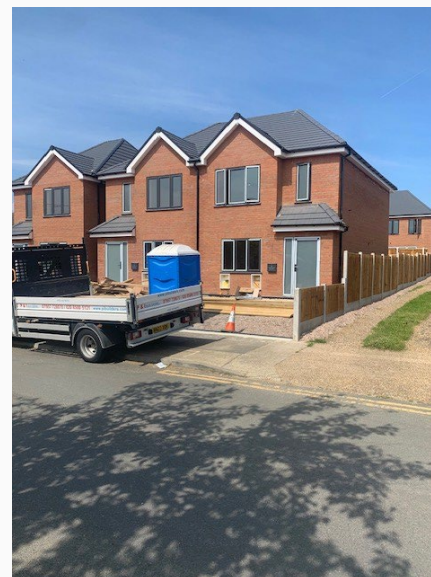
Houses recently constructed on land at Tweedway
